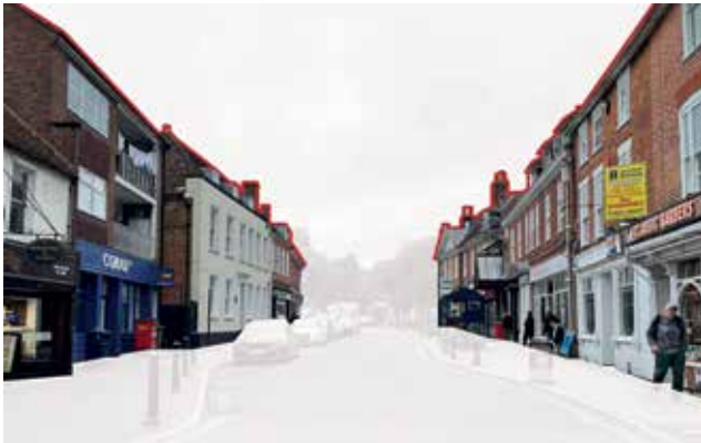
Figure 51: Roofline study on High Street showing a variety of gable arrangements and roof dormers. Building heights vary between 2, 2.5 and 3 storeys.
