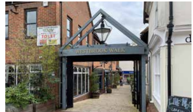
Figure 39: Westbrook Walk was created in early 1980s as a link between Lady Place car park and the High Street
