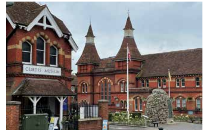
Figure 42: The Curtis Museum, at the intersection of Church Street, High Street and Normandy Street is a key landmark.
