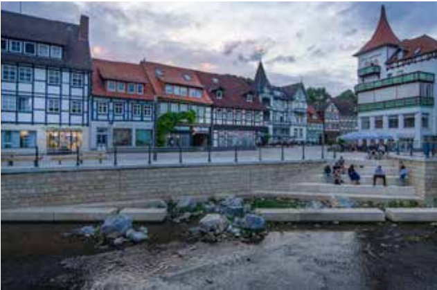
Figure 85: Creating access to existing waterways
