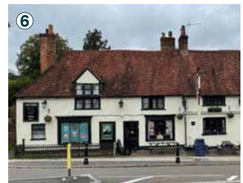
The White Horse public house, Grade II listed.
