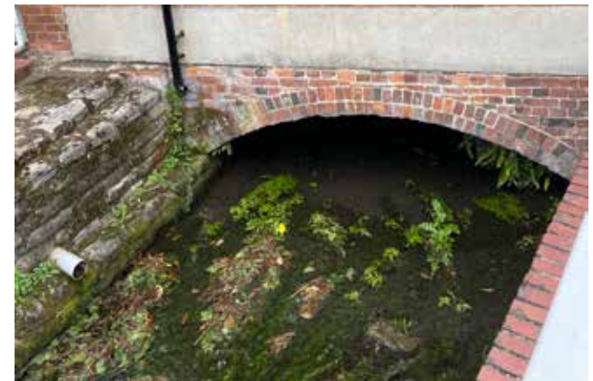
Figure 67: Culverted River Wey
