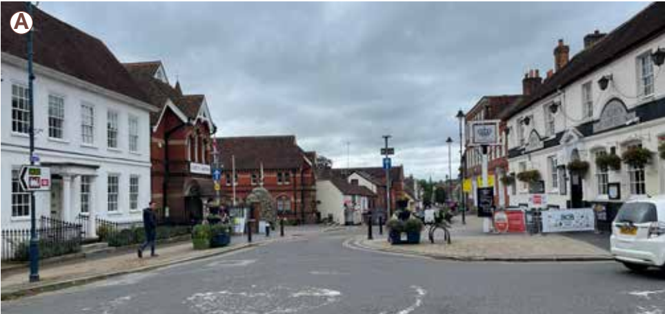
Figure 33: The intersection at Normandy Street and High Street is a gateway into the Town Centre but the public realm lets down the historic setting.
