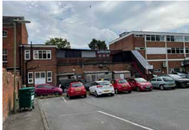
Figure 91: Area 1 - Rear view of Hamlet House and the car park
