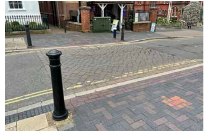
Figure 66: Example of surface treatments inconsistencies and lack of response to surrounding heritage assets.
