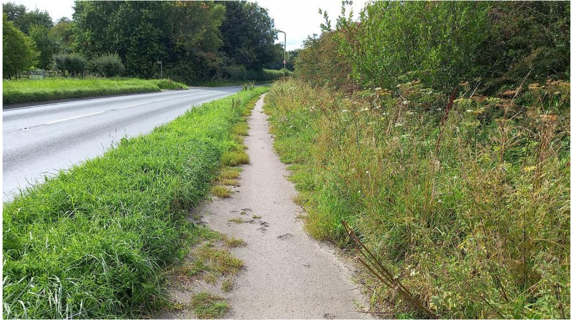
Footway alongside A339
