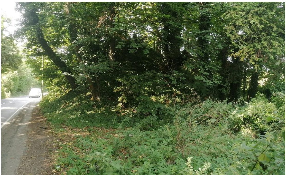
Basingstoke Road embankment
