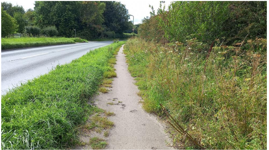
Footway alongside A339
