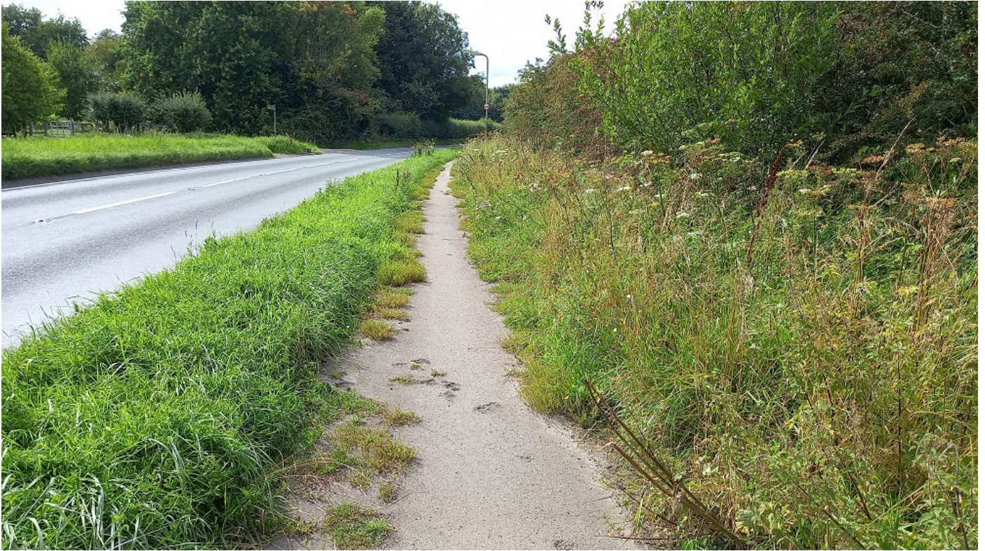
Footway alongside A339
