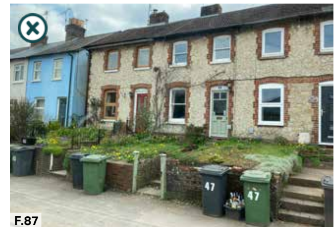
Figure 87: Positive example of waste bin storage, all bins hidden behind the boundary wall on the driveway within the plot
