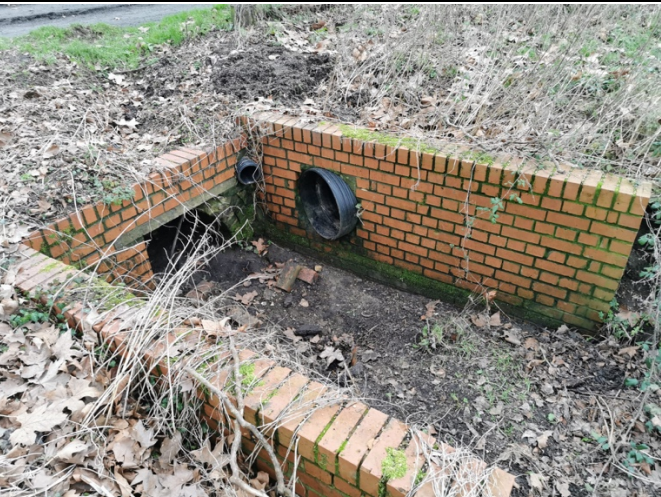
Plate 6 – Brick Kiln Lane Culvert Structure
