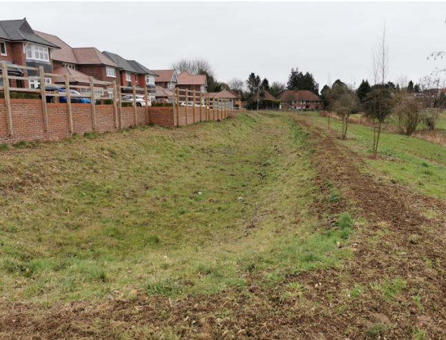
Plate 3 – SuDS attenuation pond site
