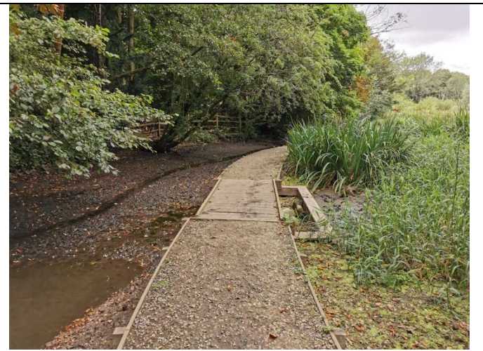
Plate 4 – Newly installed riverside raised path and recycled plastic footbridge
