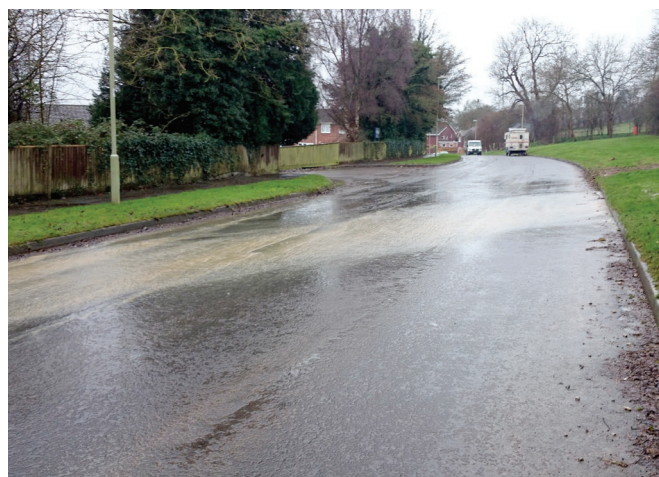
Evidence of rain water run-off leading to flooding from high ground in North Alton across Gilbert White Way
