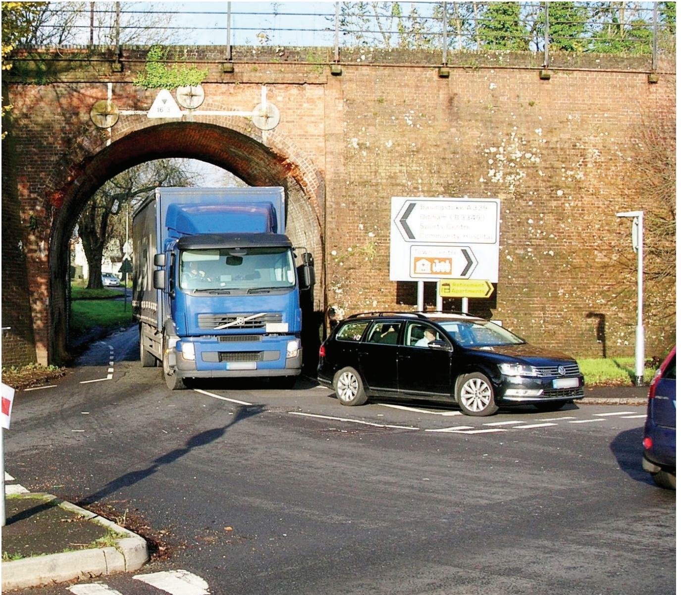
Butts Bridge – a brick arch structure.
