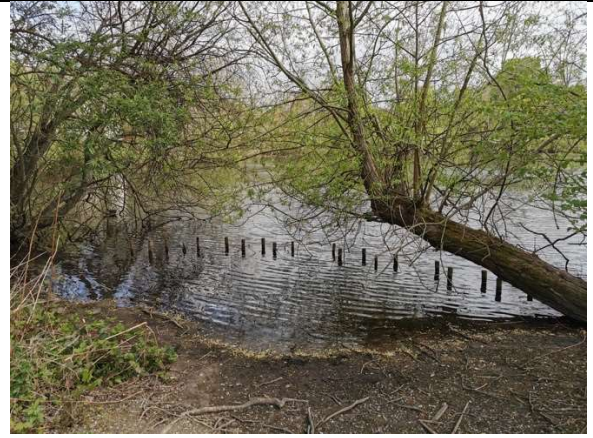
Plate 6 – Failed revetment from previous dredging operation
